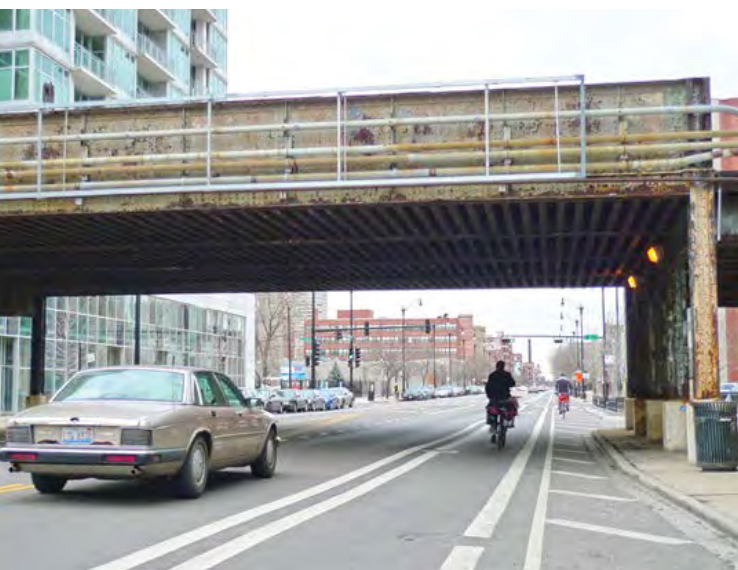
Figure 14. Buffered Bicycle Lanes on Wabash Avenue in Chicago Photo Credit: Stacey Meekins
