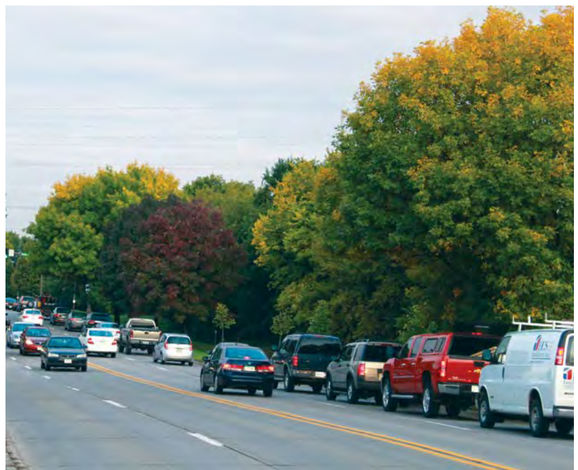
Figure 11. Four-lane Undivided Roadway Intersection Operating as a de facto Three-lane Cross Section Photo Credit: Tom Welch
