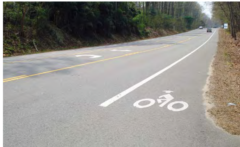
Figure 19. Bicycle Lane on Rural 3-Lane Section, Lawyers Road, Reston, VA Photo Credit: Virginia DOT
