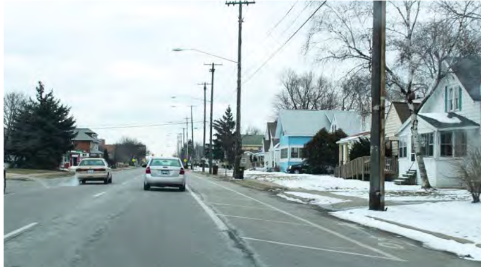
Figure 18. Painted Buffer Between Through Lane and Bicycle Lane in Lansing, Michigan Photo Credit: Jennifer Atkinson
