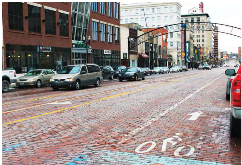
Figure 10. Road Diet in Flint, Michigan, Central Business District Photo Credit: Jennifer Atkinson
